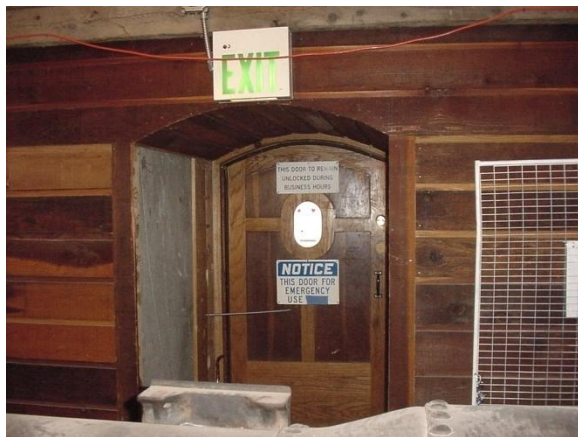
Lower level at exit door.
