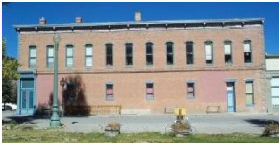
Hough Building South Elevation
