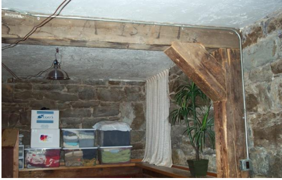
Photographs of timber reinforcement construction beneath main floor.
