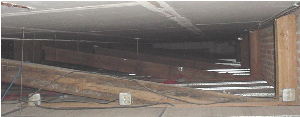
Below: Structural retrofit, showing strut and vertical column.
