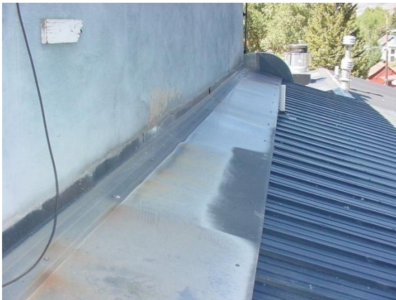
Sheet metal flashing at metal roof
