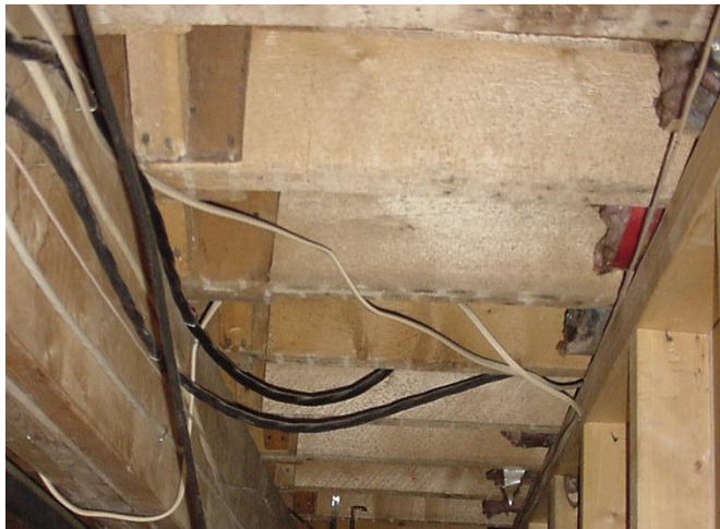
Left: 2x10 first floor framing visible at Building 2 kitchen crawl space. Note 2x6 knee wall at right.
