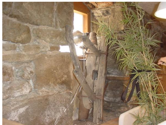
Lower level stone wall with lightwell.
