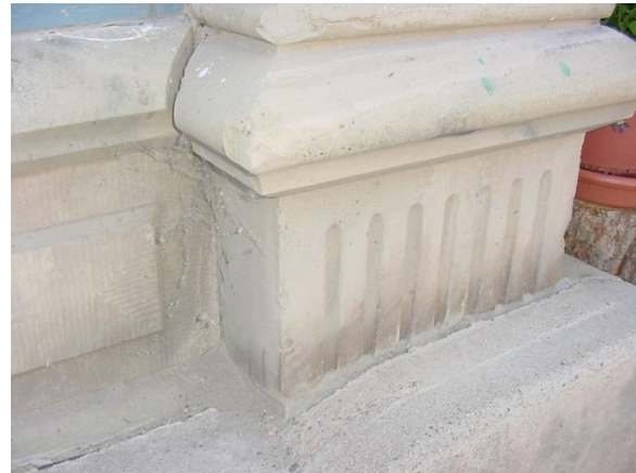
West elevation of building 2 with concrete curb at stone base. Detail at concrete curb.
