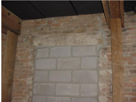
Left: Hadite cinder block behind south elevation window.
