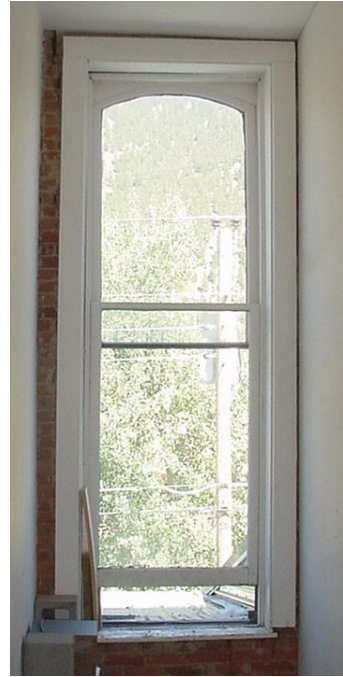
Upper level window.
