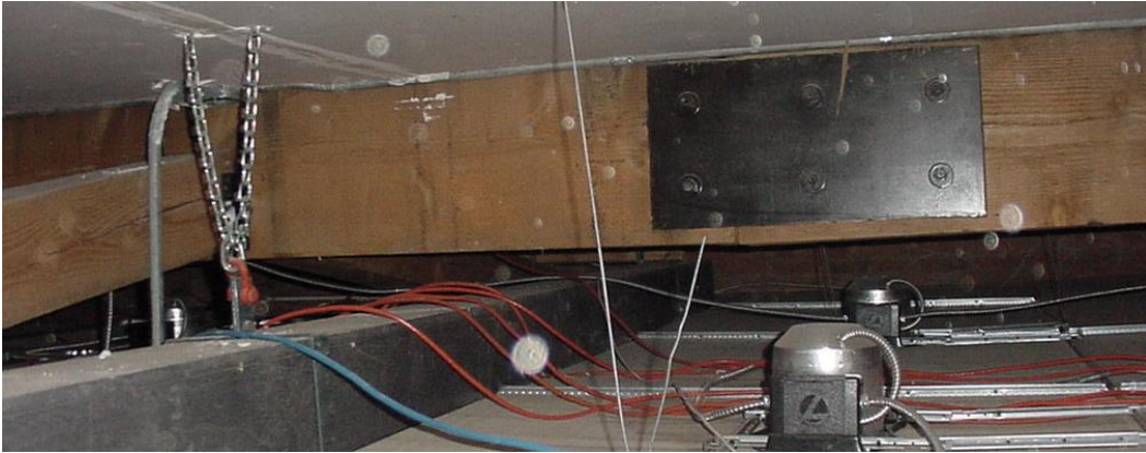
Above: Structural retrofit showing central beam, strut and horizontal member.
