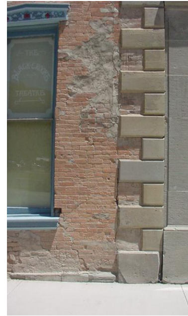
Main level detail.
