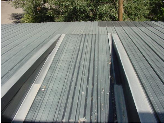
Metal seam roof at second level.
