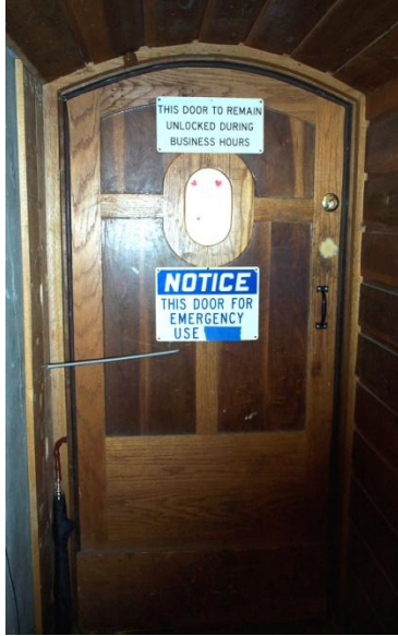
Non-original exit door from lower level. Wood, four panel with lite.
