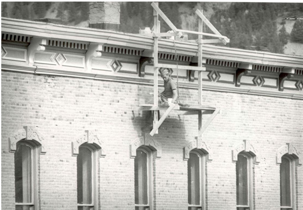
Cornice painting with makeshift scaffold. Photograph circa 1987.
