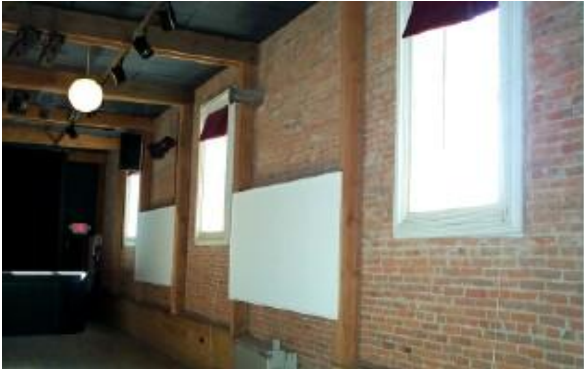
Above: Windows on south wall of theatre.
