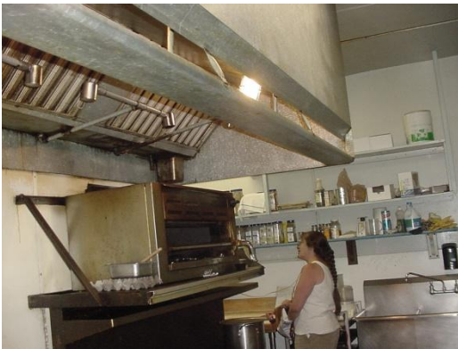
Kitchen, looking east.
