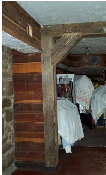
Photographs of timber reinforcement construction beneath main floor.
