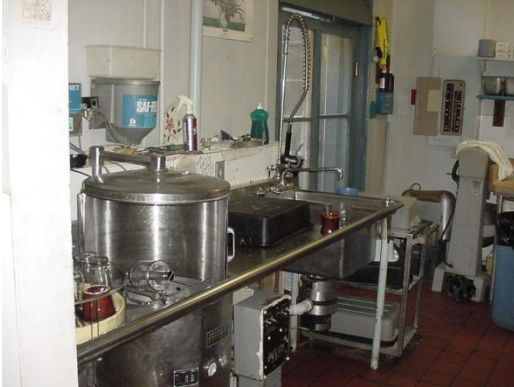
North wall of kitchen.
