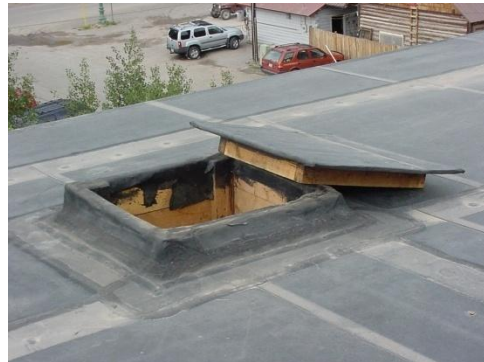
Detail at east roof hatch.
