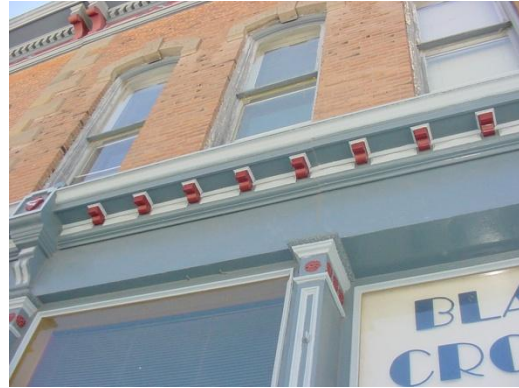
Cornice at building 1.
