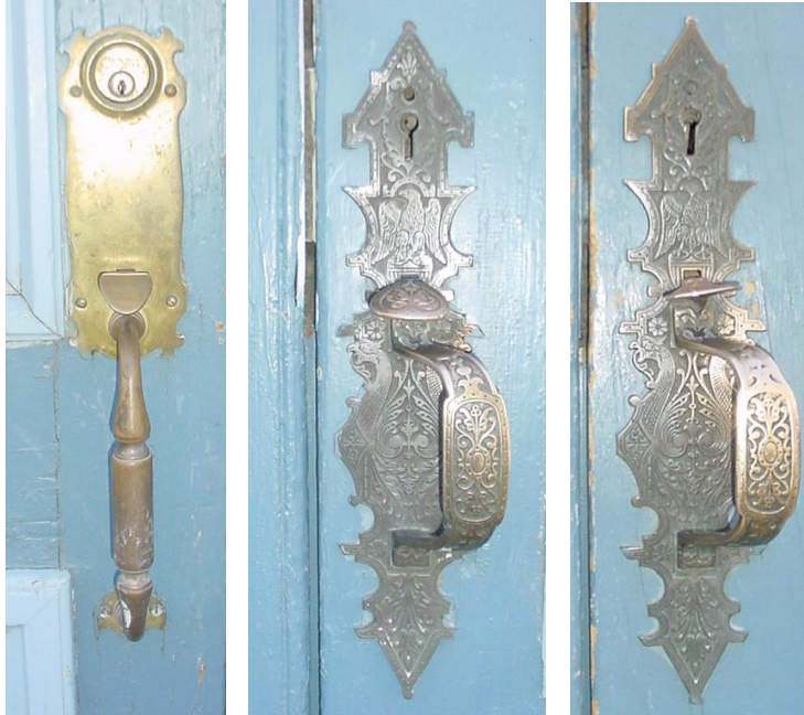
Entry door pulls: Center door, east doors.
