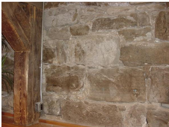
Lower level stone wall
