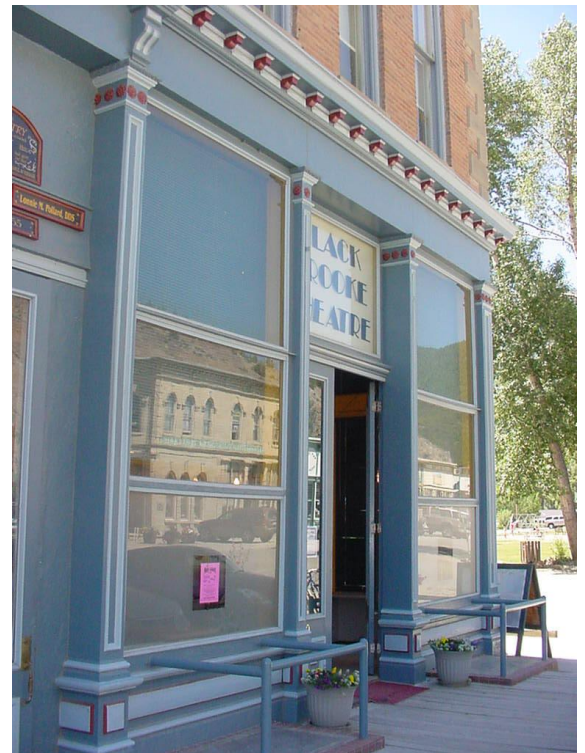
Building section 1: cast iron pilasters and storefront system.
