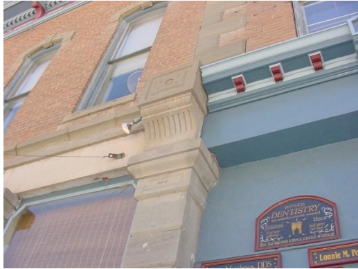
Cornice at building intersection.
