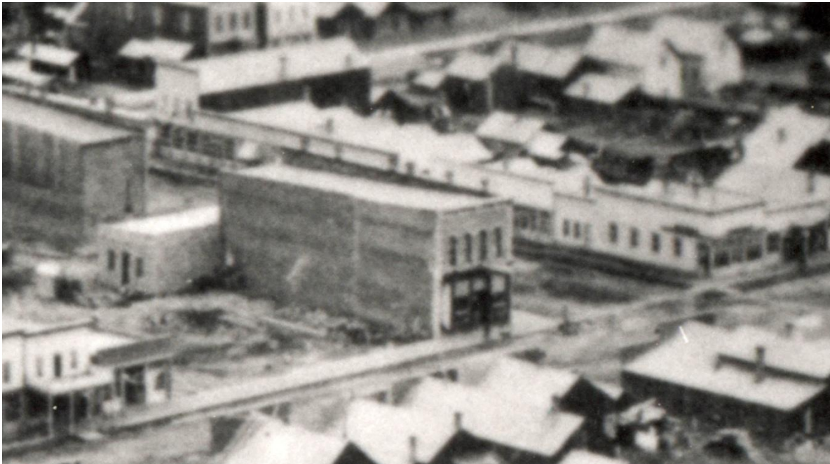
Building 1 prior to the construction of Building 2. Photograph Circa 1880.
