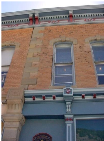
Cornice and upper cornice.
