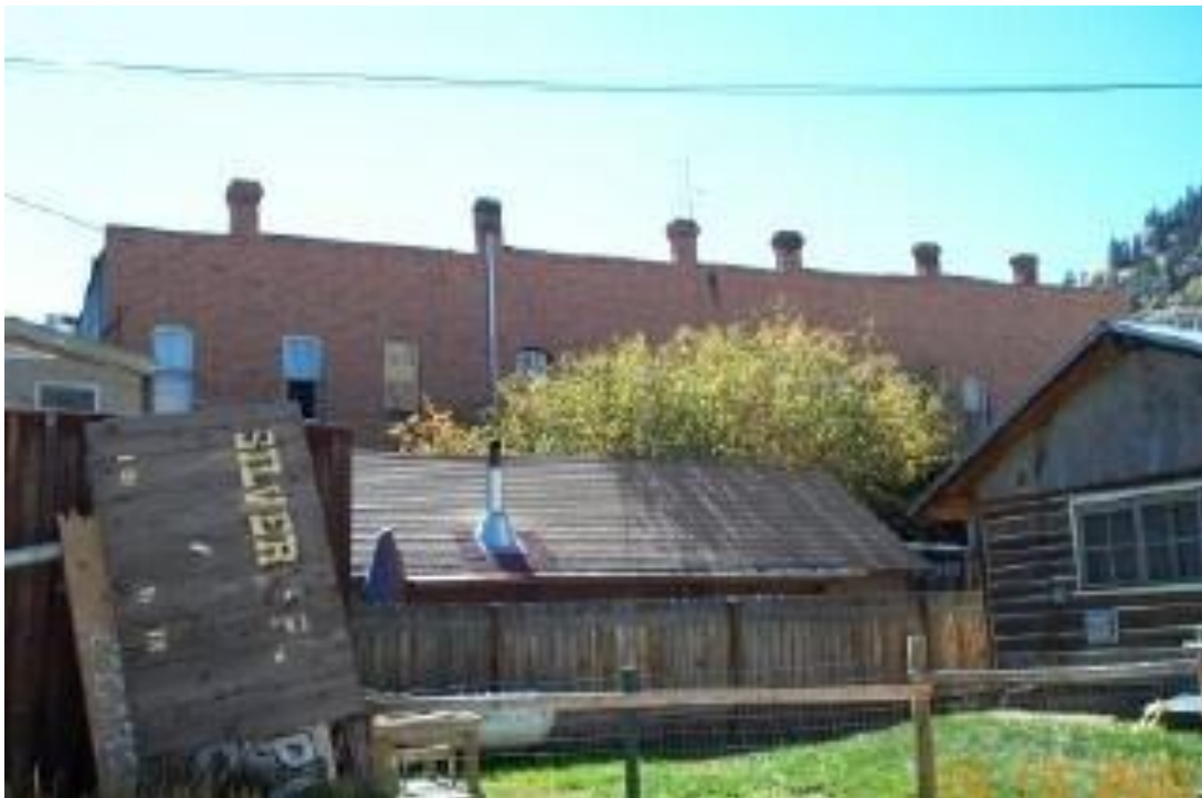
Hough Building, Building 2 north elevation (partially obscured by adjoining structures).
