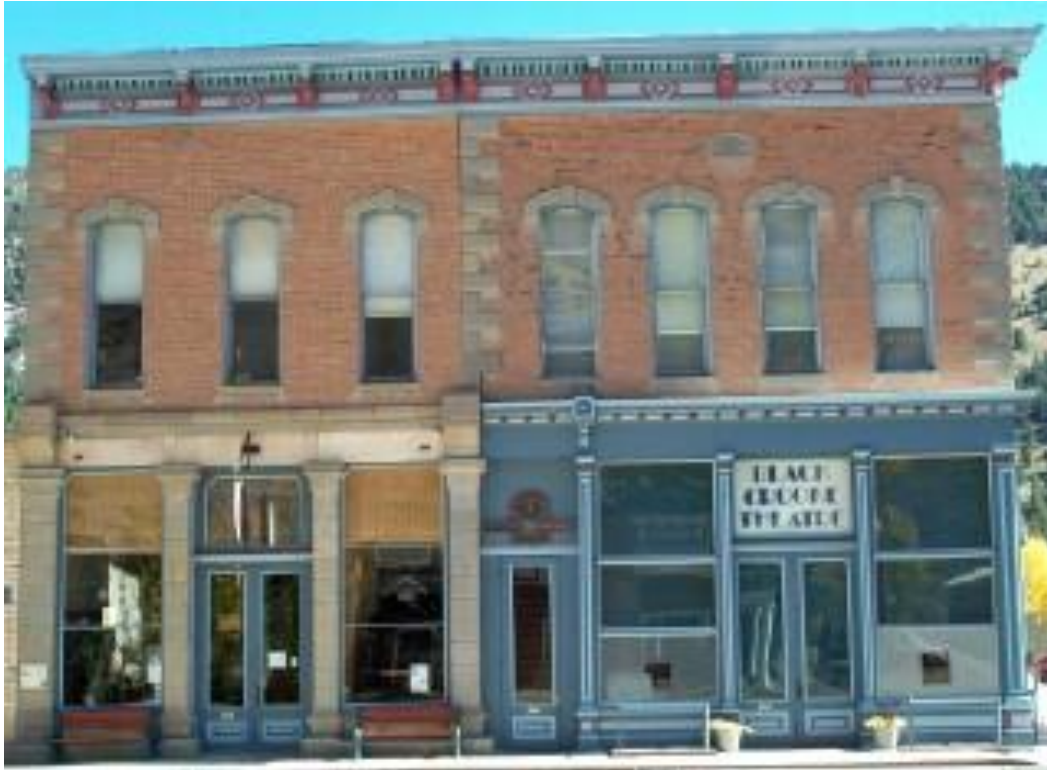
Hough Building West Elevation
