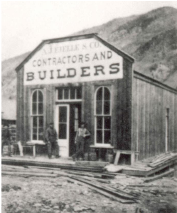
A. J. Fielle & Company Contractors and Builders
