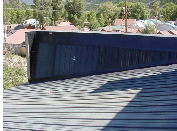
Metal seam roof, looking south.
