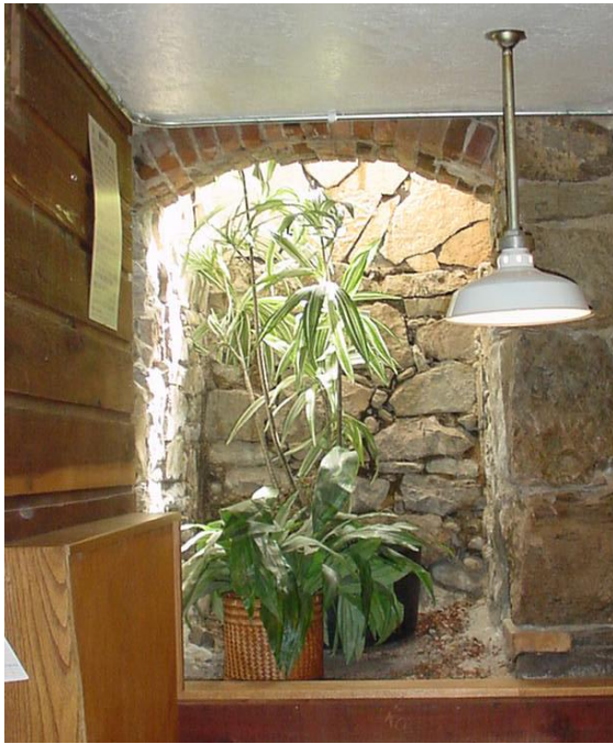
Lower level lightwell.
